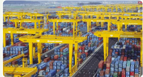
Automated RMG Crane (ARMGC)
